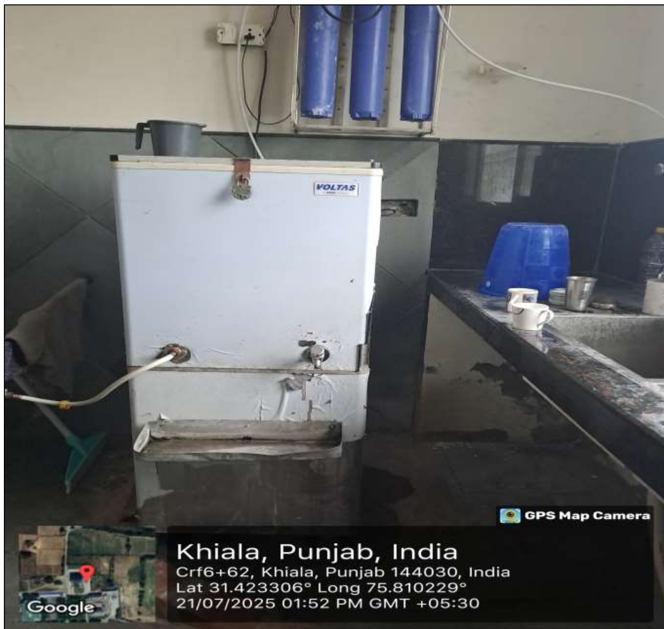
Existing RO Filter connected with water cooler in Campus
